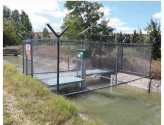
Irrigation Channel Samsun-TURKEY
