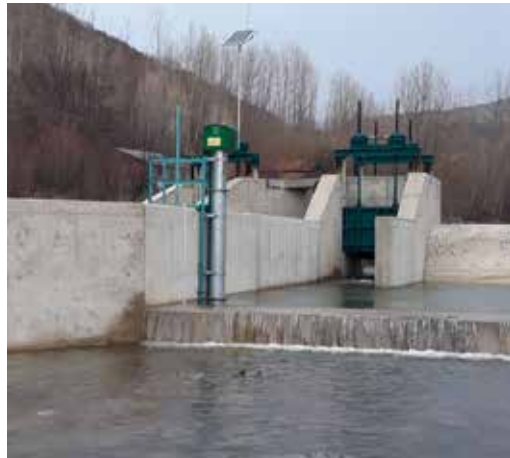
HPP Water of Life Station-Trabzon
